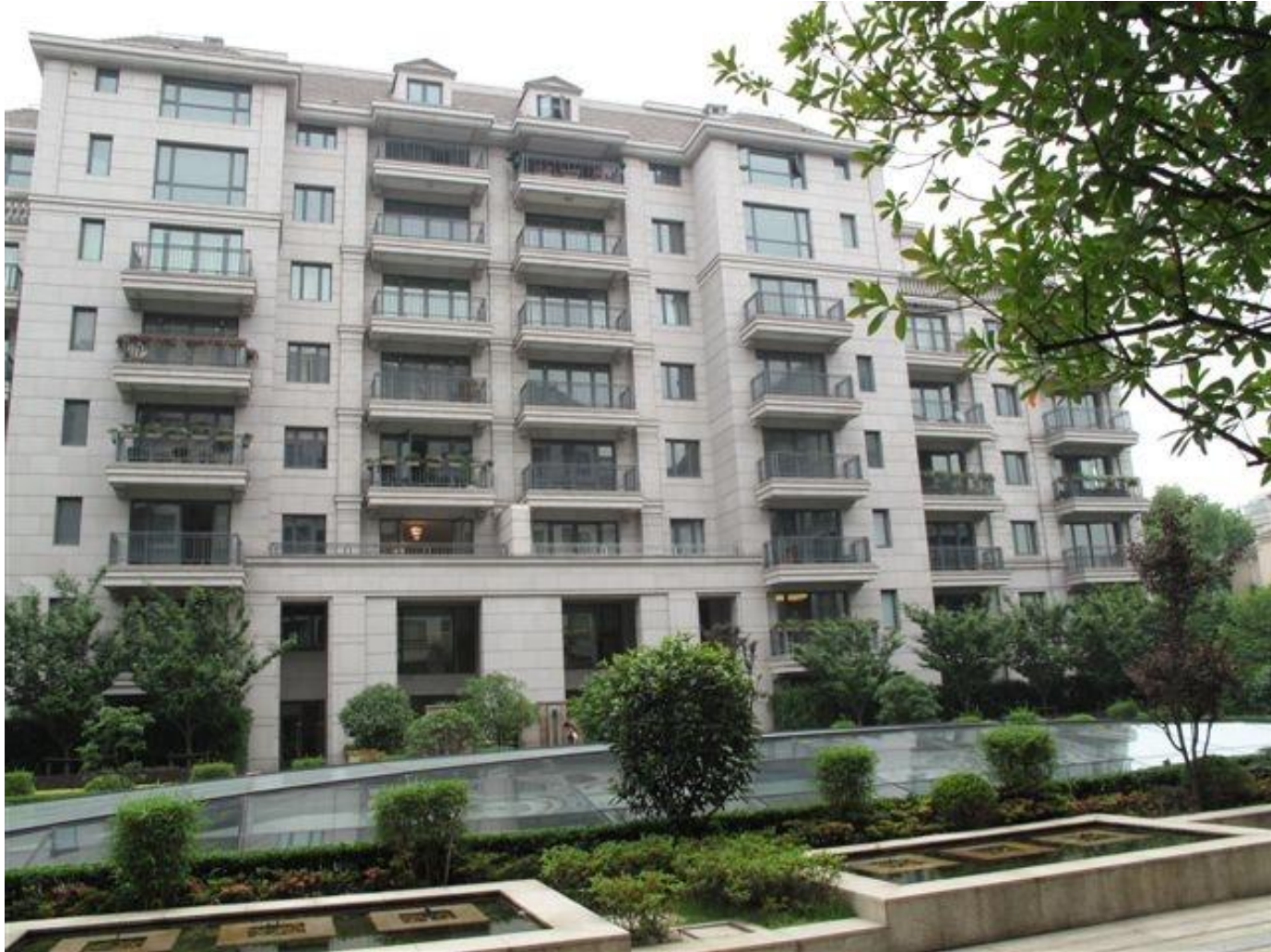
Main building with central courtyard/covered indoor pool
