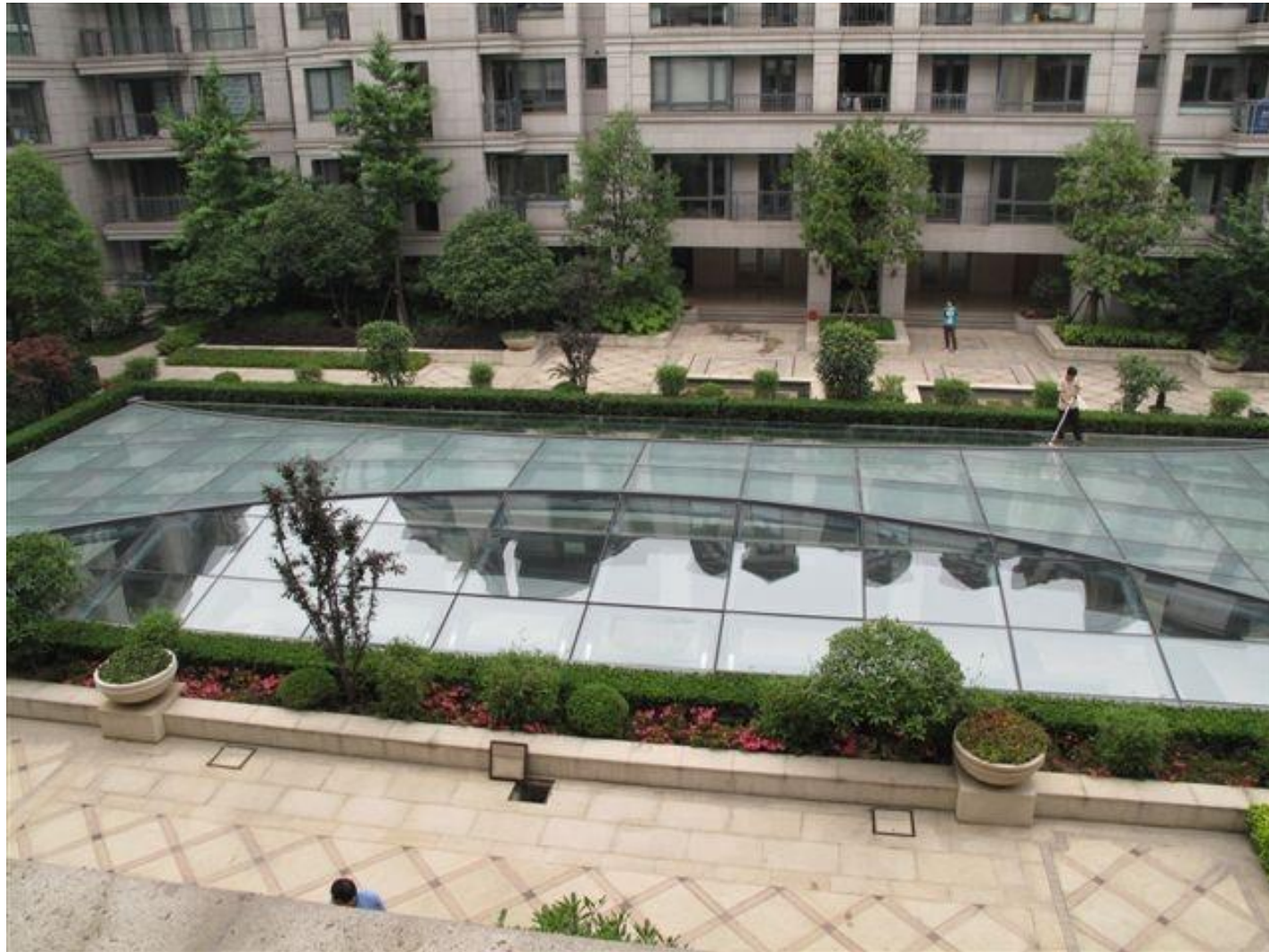
Central courtyard/covered indoor pool
